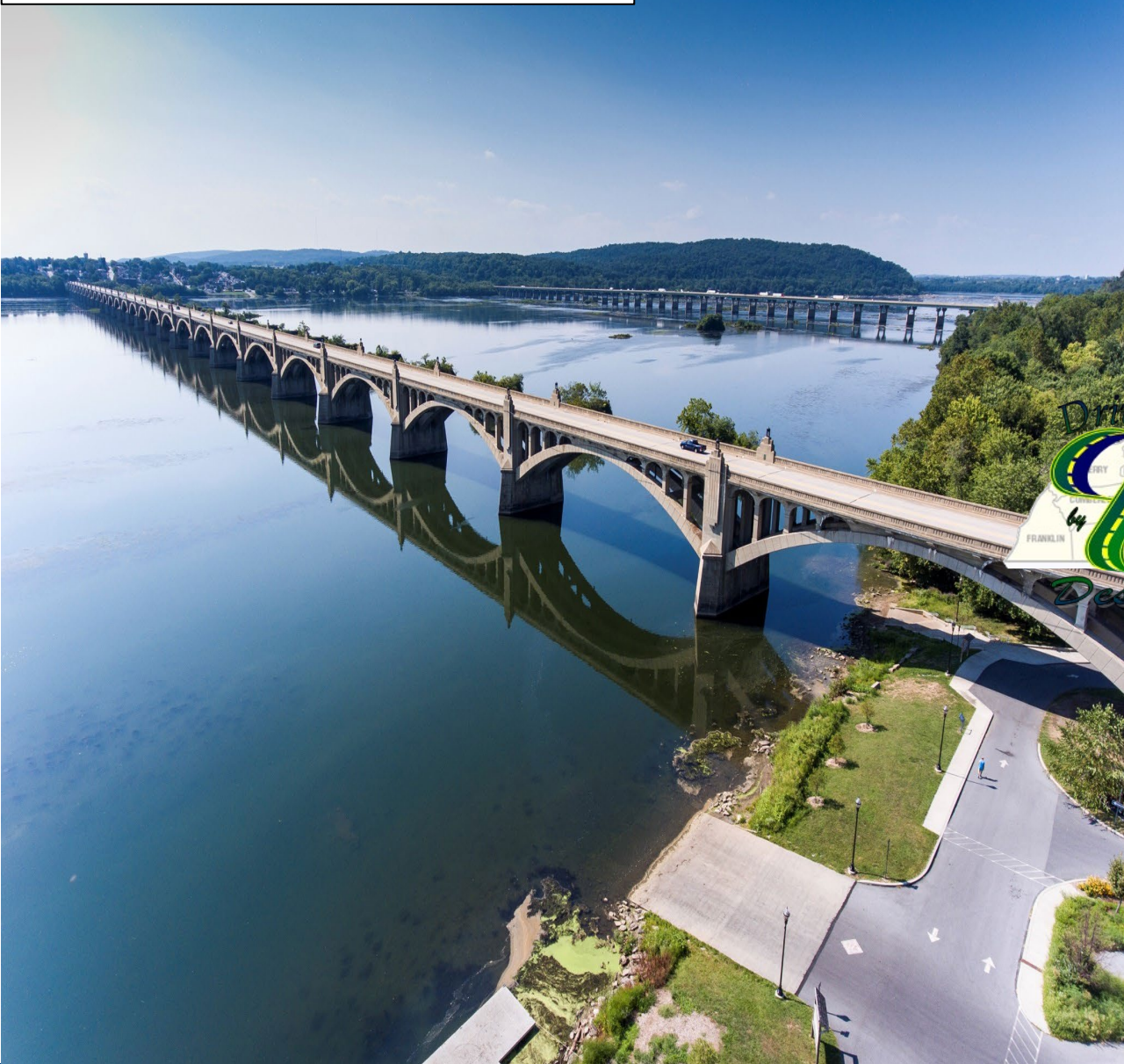
Columbia/ Wrightsville Bridge – Late 2026
