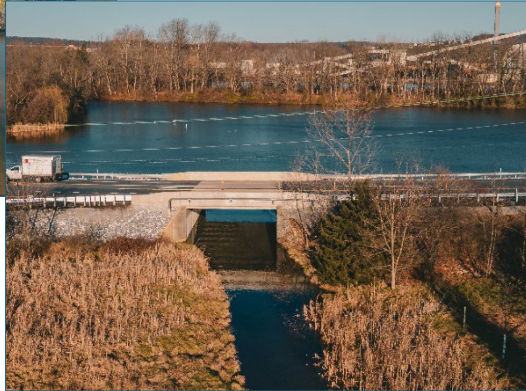
York Road Bridge
