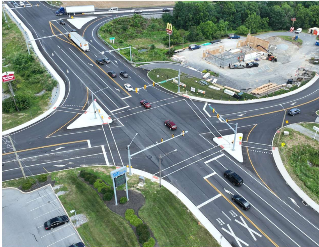
Centerville Road Interchange
