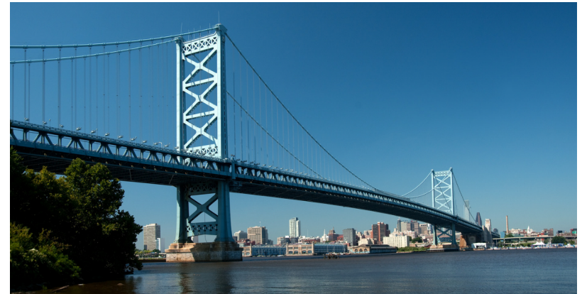
Long Span Bridges: L > 250 \text{ ft} (approx.)
